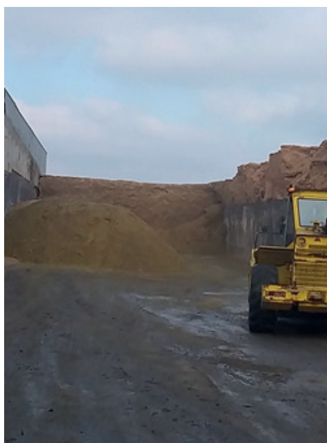
Picture 1. Biogas plant feedstock area, original source N.R. 2019.
